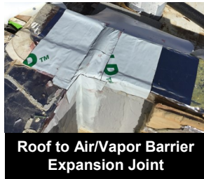
Vertical Expansion Joint
