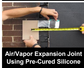
Expansion Joint at Existing Building
