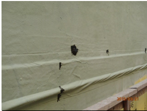
Horizontal Expansion Joint
