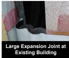
Roof to Air/Vapor Barrier Expansion Joint
